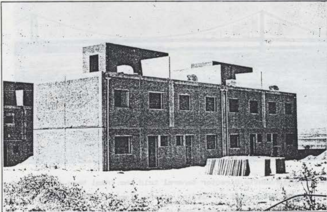
More pre-fabricated housing units are being built
